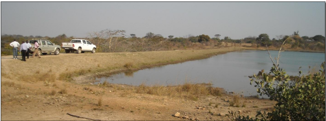
PHOTO: Small dam, Chongwe, Zambia. Copyright © 2011 Franz Hollhuber
