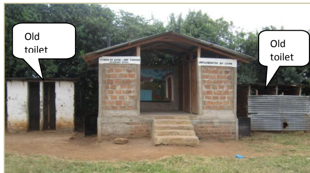
ECOSAN toilet in Bar Mathonye Primary School with old facilities by the sides
